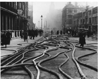
Water delivery is expressed in terms of DELIVERY PUMPS – which is the number of hoses that can be supplied by a given appliance.
